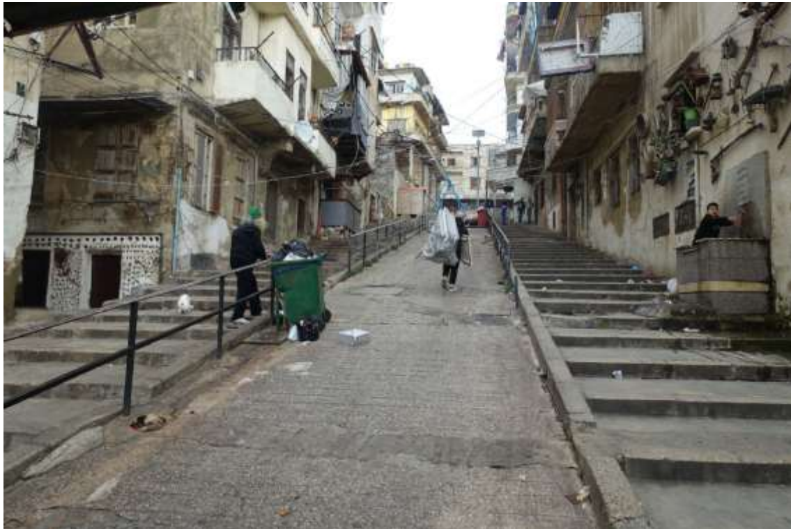
Selected stairway for pilot intervention 34.4337851, 35.8477734
