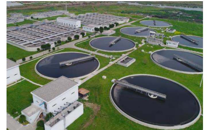
Fig.4: Mersin wastewater treatment plants. Source: Mersin
