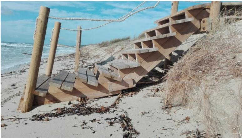
Beach access stairs undermining due to wave-induced erosion at Son Bou beach (November 2018)
